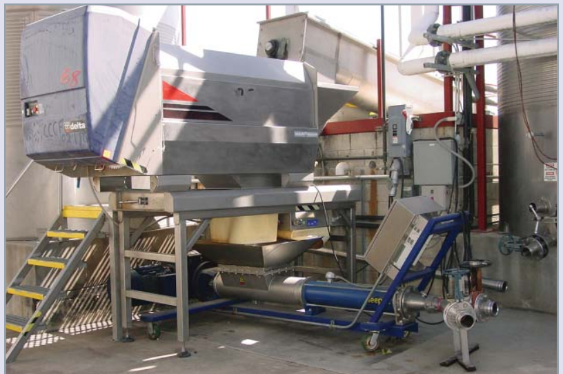
Final installation of the Seepex Pump below the Delta8 Crusher
