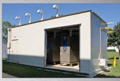
The project above includes a unique Fulton custom-built enclosure for four Pulse® boilers. While the enclosure is served by exterior pumps, a fully-functioning hydronic boiler system complete with supply and return piping, ModSync® sequencing system, control valves, expansion tank, intake air and exhaust flues made for a simplified "plug and play" installation.
