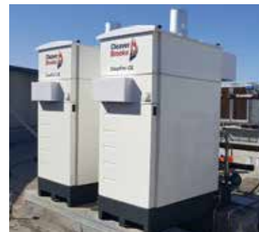
CB Hot Water Boilers for Sacramento Facility
