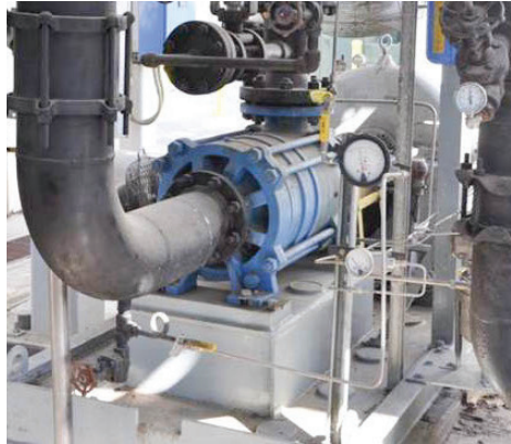
BOILER FEED PUMP PACKAGE
