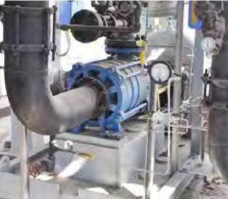
BOILER FEED PUMP PACKAGE
