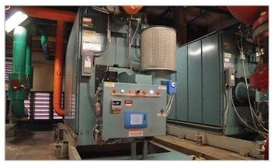
The new CB ProFire MTH Burner and control panel on one of the boilers
