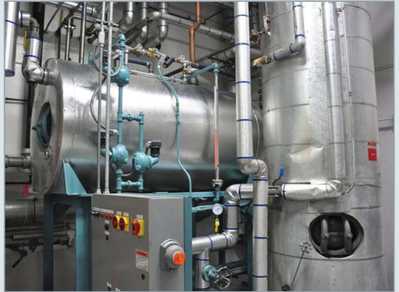
Finished installation of new feed tank.
