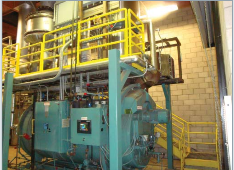
Finalized boiler installation
