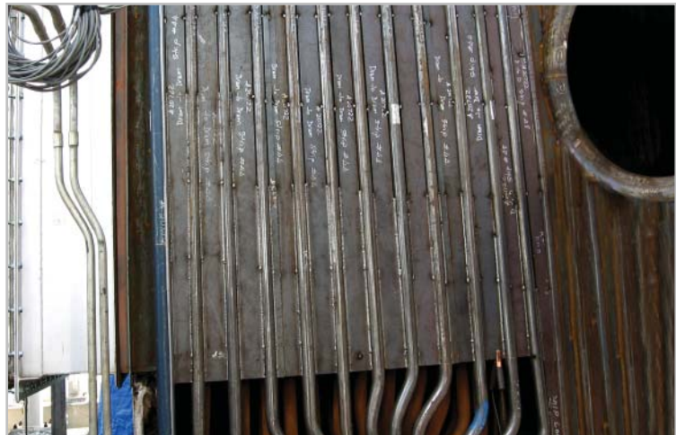
The completed section of tube replacement for the boiler front wall
