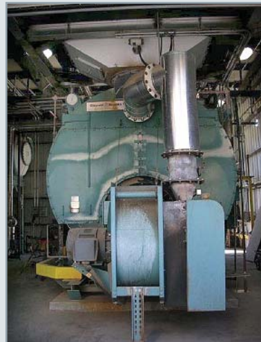
Final installation of the new boiler
