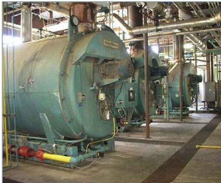
Three existing boilers were retrofitted to meet lower NOx standards
