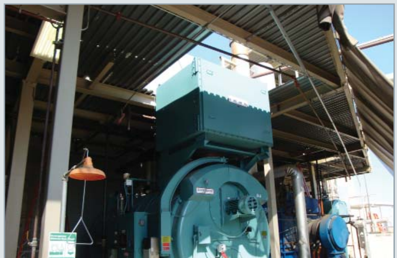
The new boiler unit with condensing economizer during construction
