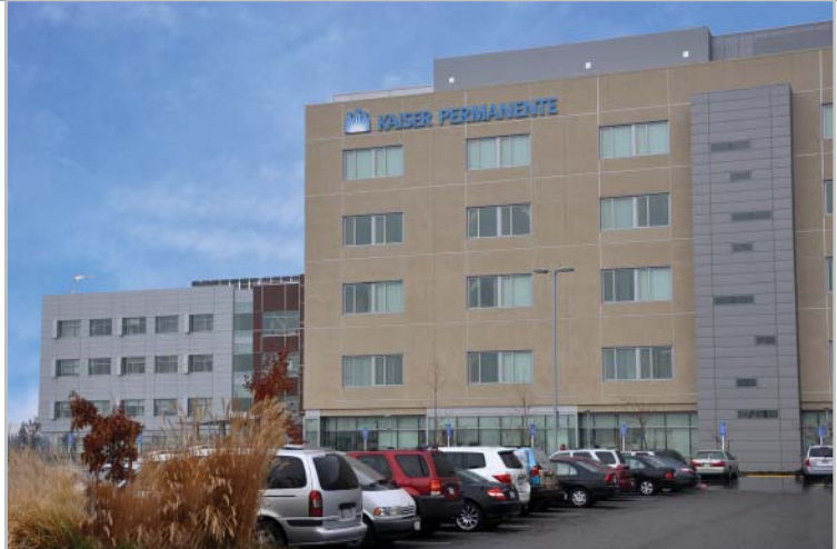
The new Kaiser Permanente Hospital located in Modesto
