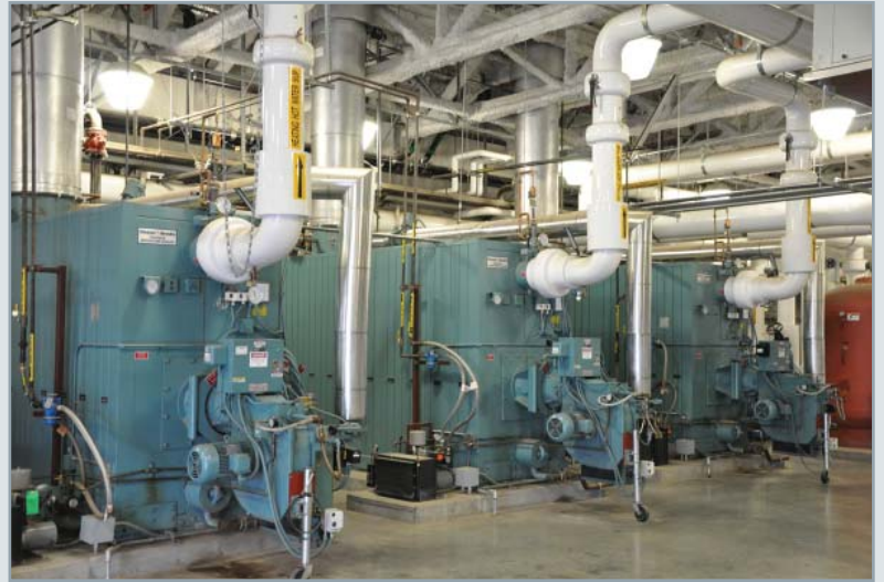
Final installation of the boiler plant
