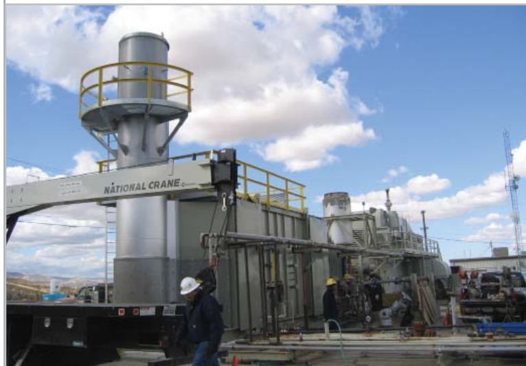
Equipment delivery and site installation in process
