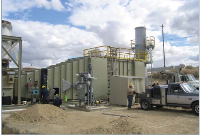
The SCR facility during installation and testing
