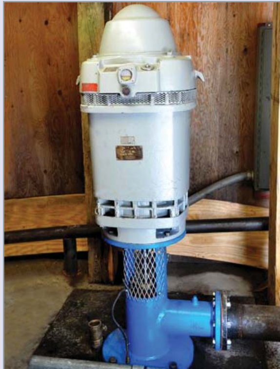
Final installation of the vertical pump
