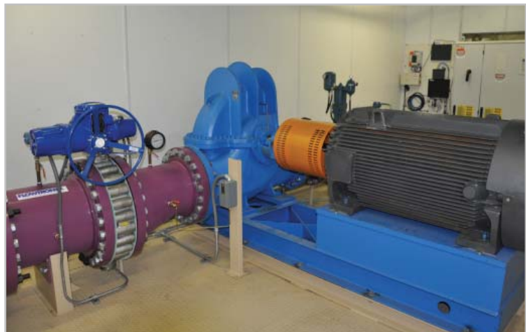
The entire pump setup featuring a Goulds Split Case 3409
