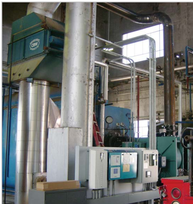
Installing the new Ultra Low-NOx burner and controls
