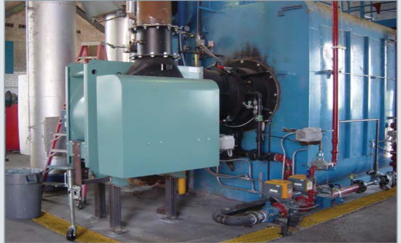
Final stages of testing and operation
